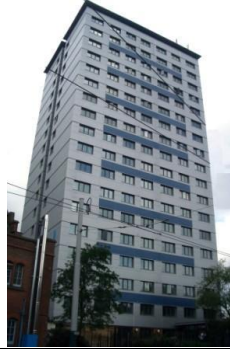
a block of flats
